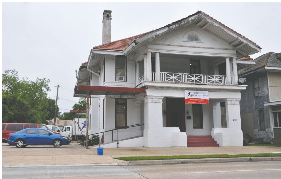
The Shreveport Center at 452 Stoner - needing some restoration.
